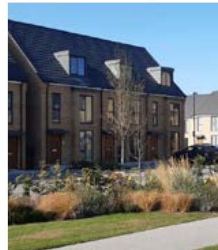
Cable Wharf, Northfleet
